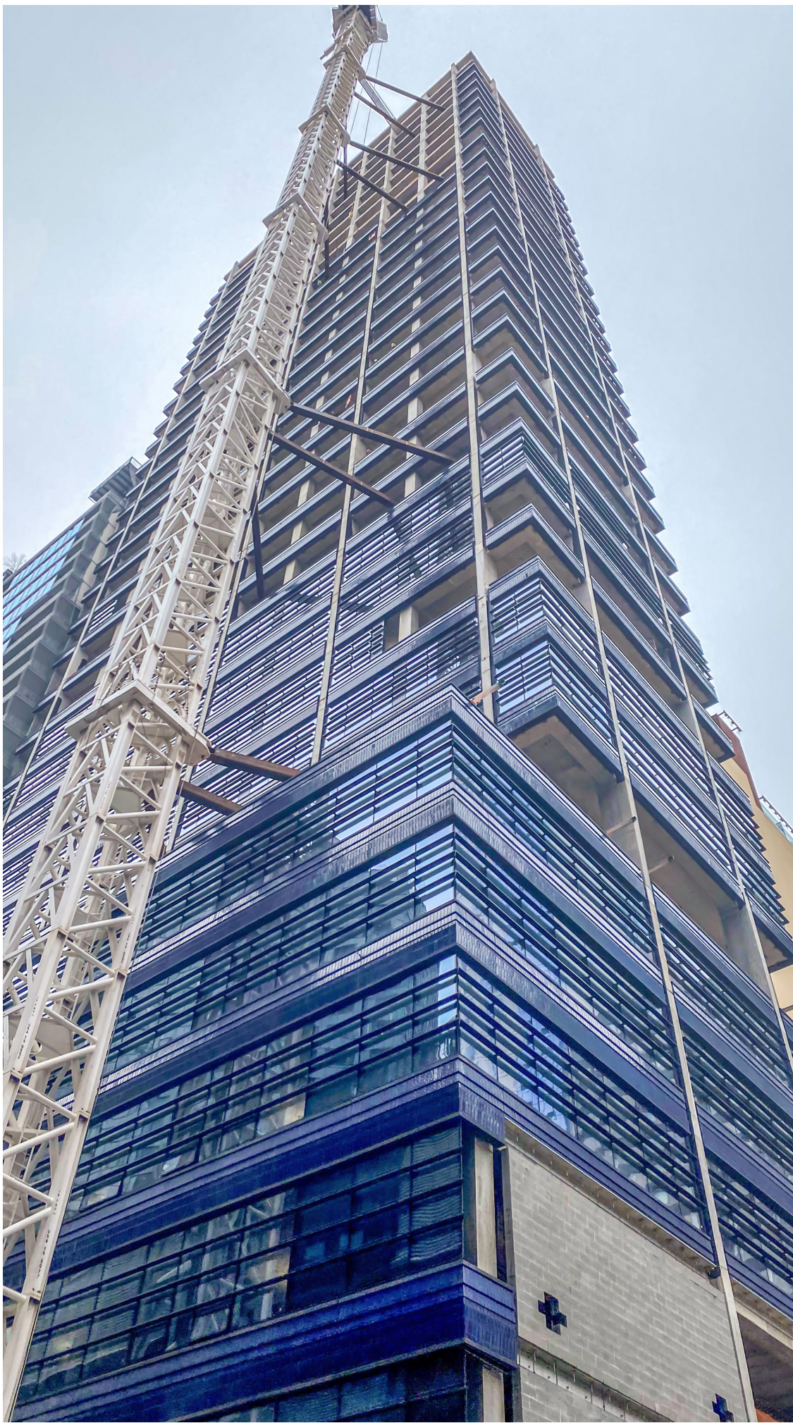
North-East corner of completed concrete structure, with ongoing precast panel and window wall facade installation.
