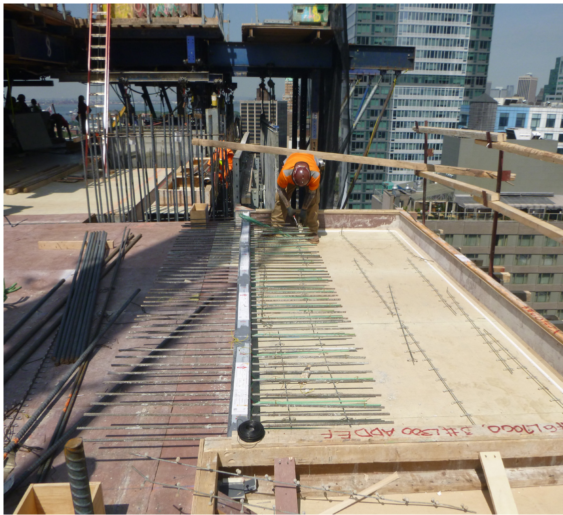
Installation of thermal bridge at cantilevered balconies
