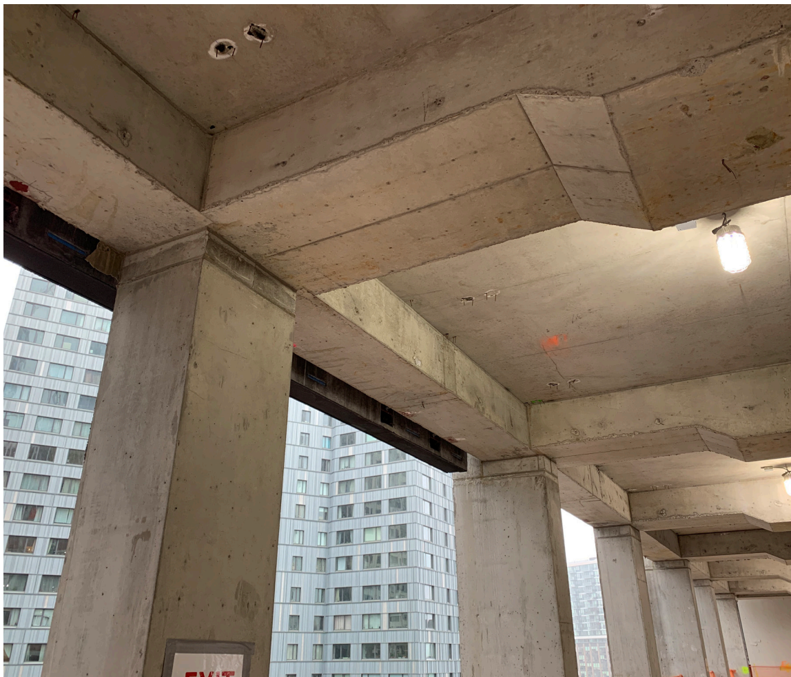
Tapering of long span beams at perimeter for integration of mechanical ducts.
