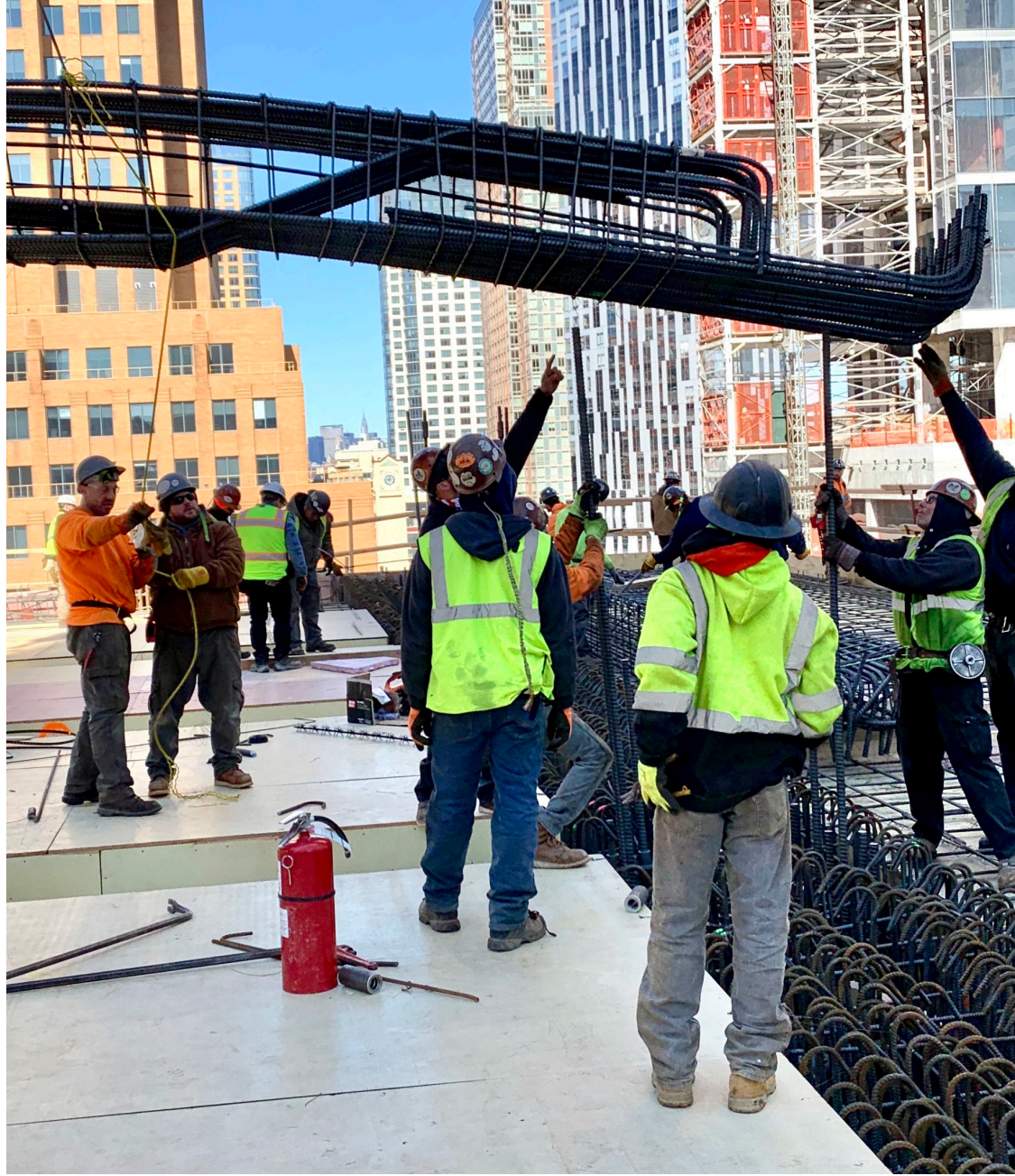
Installation of long-span beam rebar
